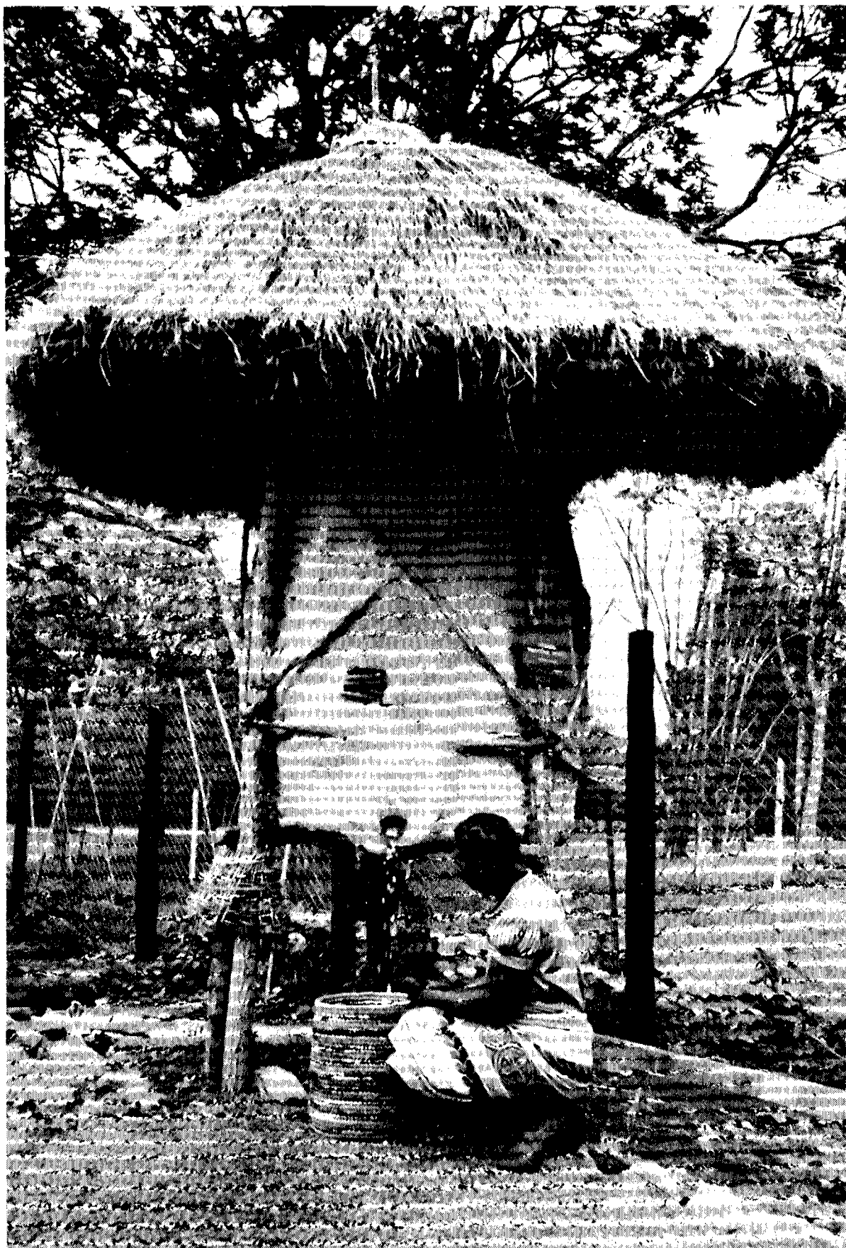
7. Improved Traditional Silo. Dry and pest-proof storage for threshed grains.
