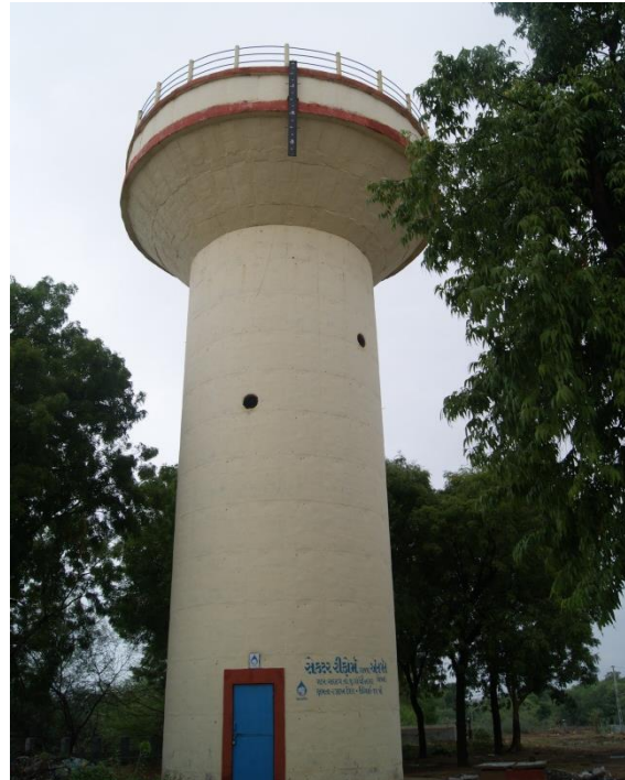
Photograph: Infrastructure built from the 90-10% contribution
