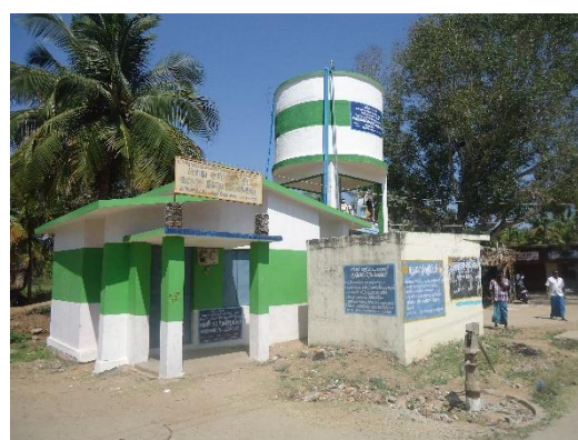
Photo 4 Renovated overhead-tank behind disused handpump in Vagurappampatti
