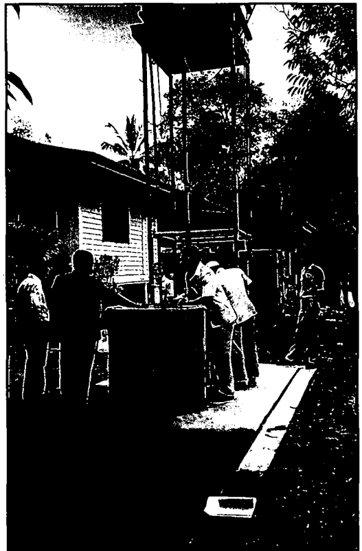
RIGHT: Typical pumped shallow well with overhead tank, rural Malaysia
