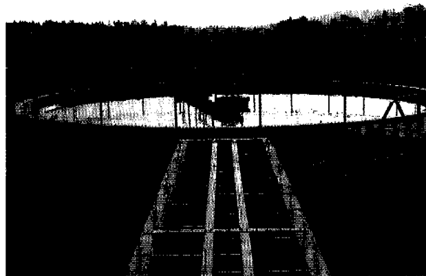
Secondary settling tank at Mitchell's Plain.
