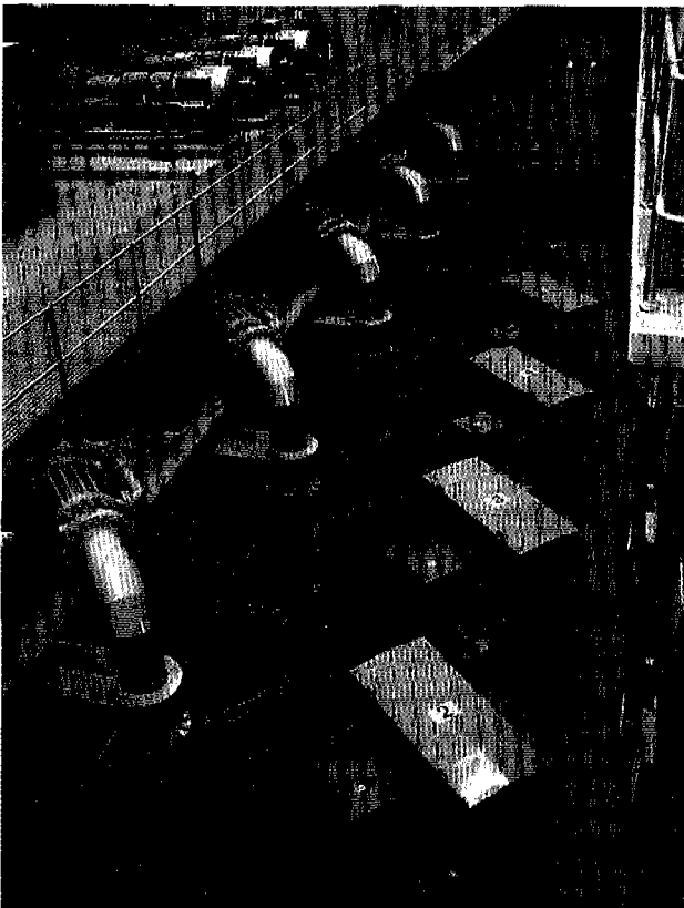
A view of the recently inaugurated high-lift pump station at the Vaalkop Water Treatment Plant of Magalies Water.
