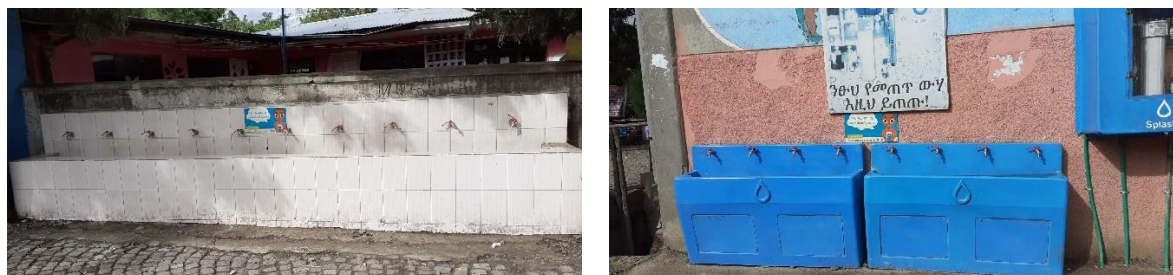
Figure 7 First generation (left) tap stands and second generation (right) - Edgat Besira primary and KG campus
