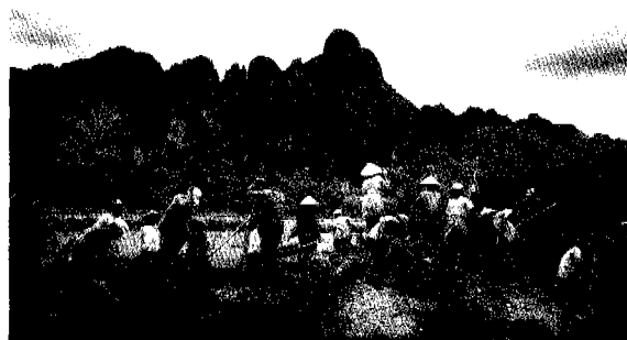
Digging the irrigation canal in Vieng Xai
