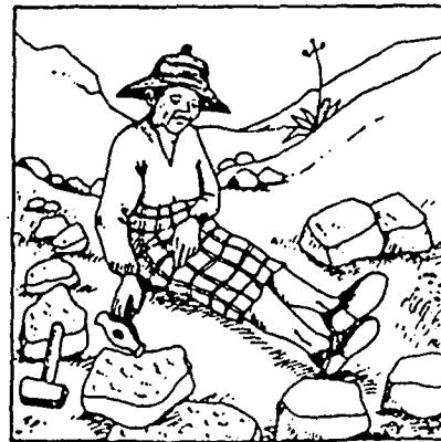
Stones to be used for building the tanks must be carefully shaped.
