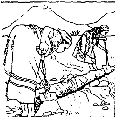
dig furrows for the pipes hard work
