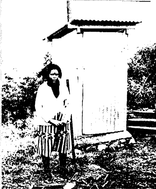
Mateboho Monnanyane, one of Lesotho's most prolific latrine builders, with an example of her work.
