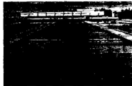
After flocculation the flocs will settle down if the water is left to rest long enough, with as little turbulence as possible. The sedimentation basin has to be large enough to give all flocs a chance to settle.
