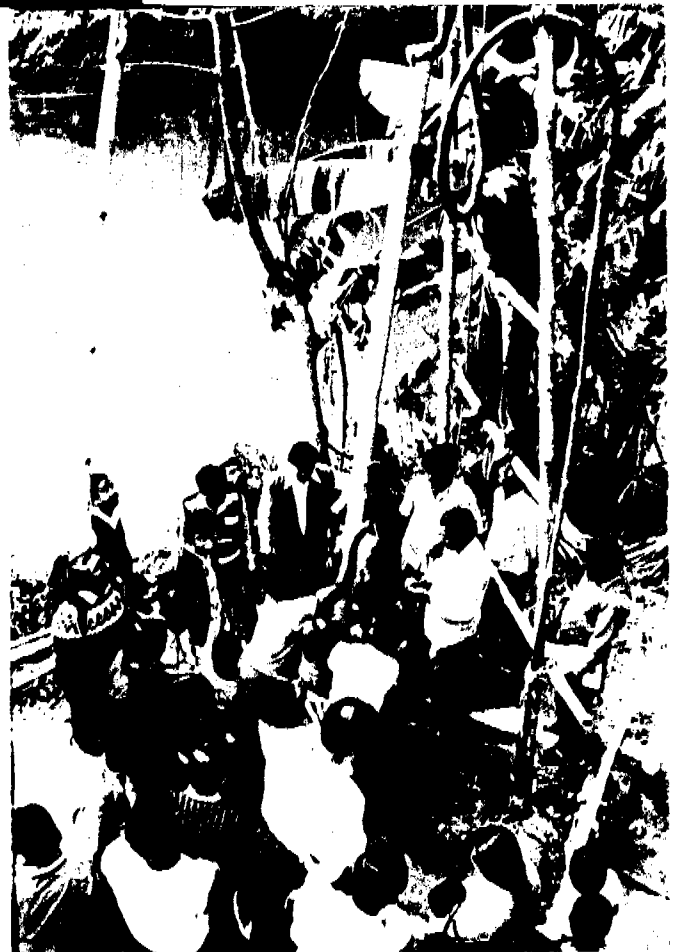
TARA HANDPUMP INSTALLATION AT SINGUR
