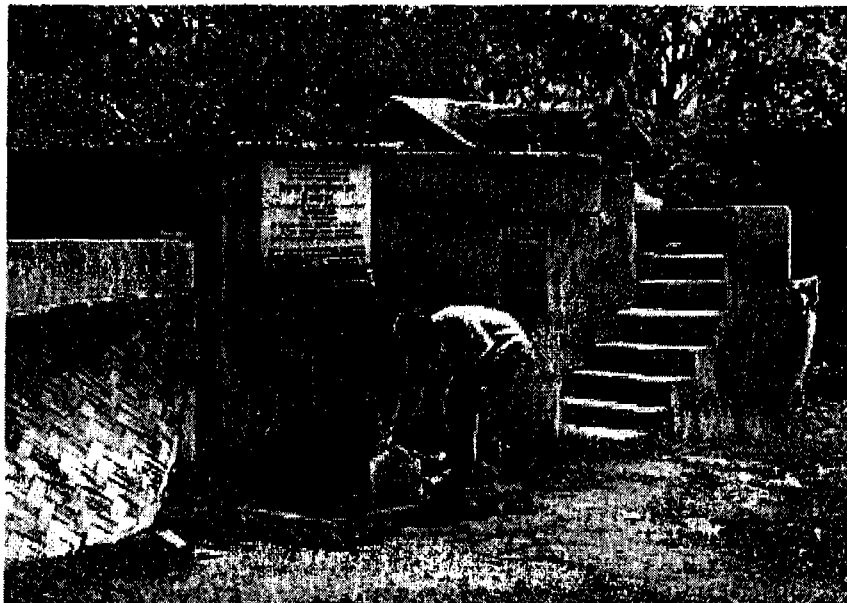
Figure 3. Village level Alum/Iron dearsination plant as developed by the All India Institute of Hygiene and Public Health.
