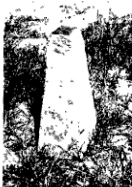
Fig. 50 A benchmark indicates the location of an approved borehole.
