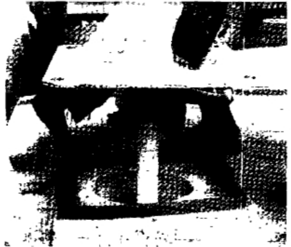
Fig. 130. A flexible gasket under the foot plate seals off the well completely
