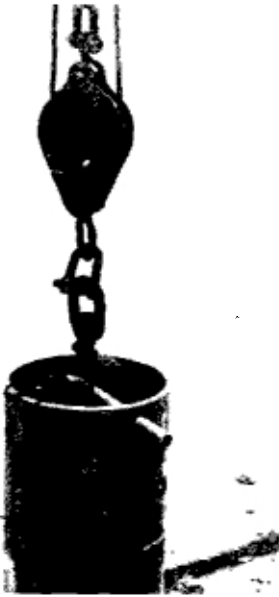
Fig 168 The casing hanging from the hook. Note that for this heavy job both pulley wheels of the upper block are used (compare with Figure 159).
