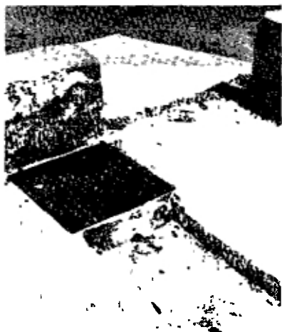
Fig 137 During repairs the well must be covered
