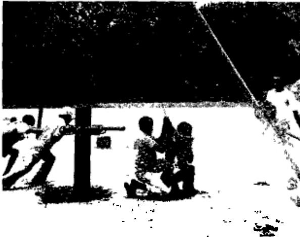
Fig. 72 While the bailer is lifted, the casing is pushed further down into the borehole.
