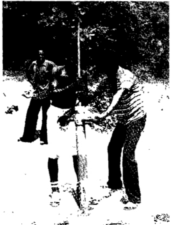
Fig 48 The casing has to be lowered while bailing and is rotated clockwise
