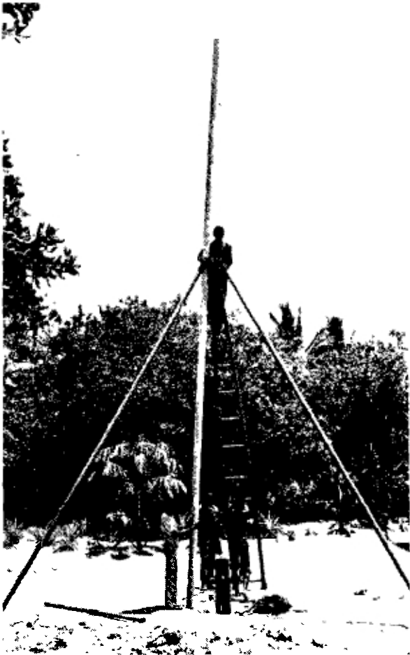
Fig. 85. The filter pipe erected along the tripod, ready for installation.
