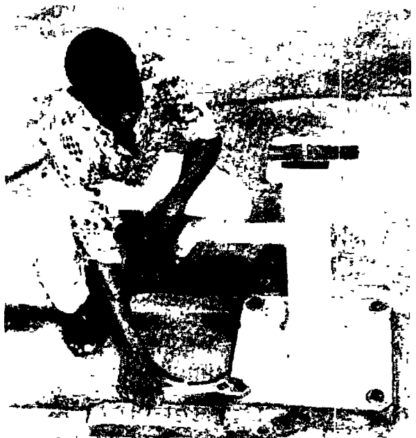
Fig. 130. A flexible gasket under the foot plate seals off the well completely
