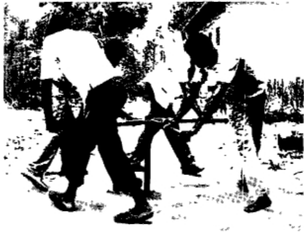
Fig. 45 If the soil is too hard, the heavy-weight set can be used.
