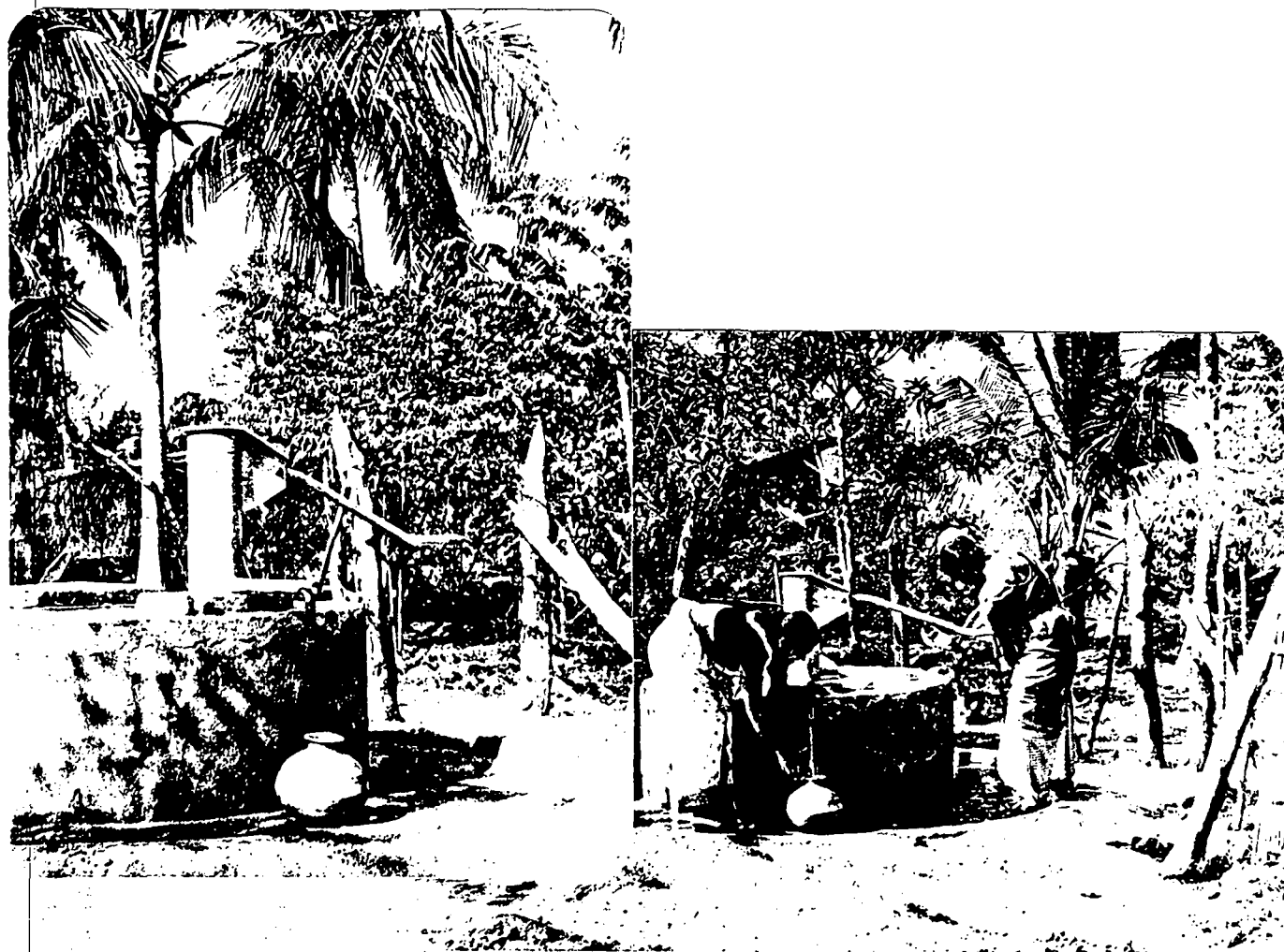
Shallow dug well and SL 15 handpump installed at the outskirts of Anamaduwa/Puttalam district, February 1988
