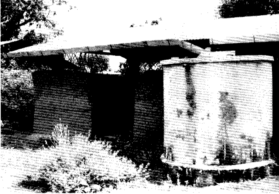
Figure 5.2: Rooftop catchment structure, which could be used for housing
