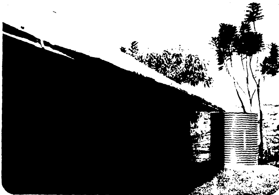
Fig. 30 A permanent house with corrugated iron roof without gable has a gutter on one side of the roof such that not all the water is collected to the ribbed galvanized iron-sheets tank in Gusii District, Kenya.
