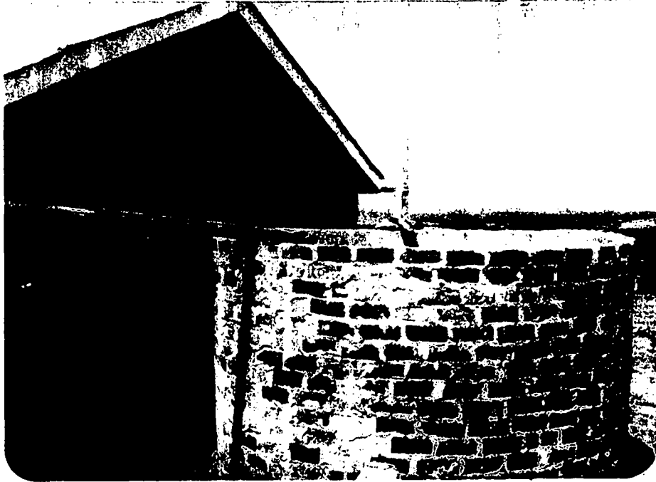
Fig. 41 The brick built tank is not sealed at the top such that dust and other impurities could easily get into the stored water in this primary school in Cusii District, Kenya.
