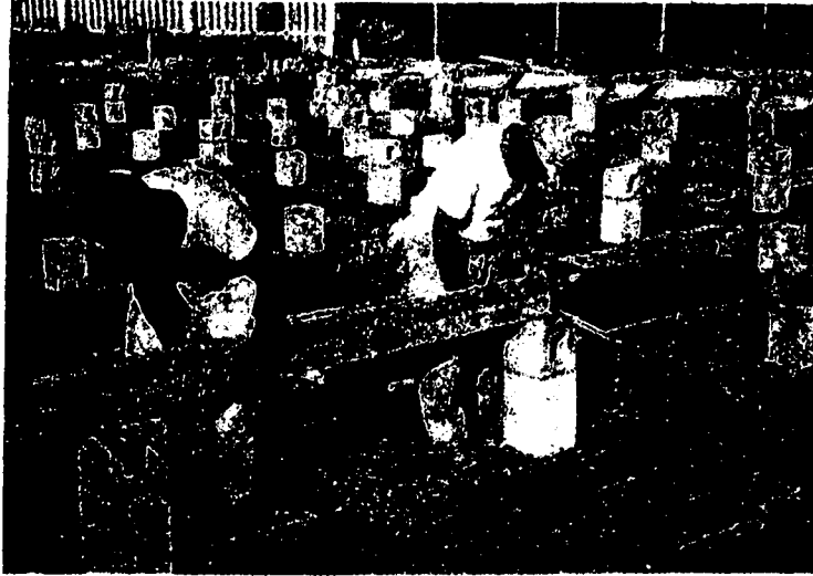
FIGURE 51. PLACING PRECAST CONCRETE BEAMS ON CONCRETE-BLOCK PEDESTALS
