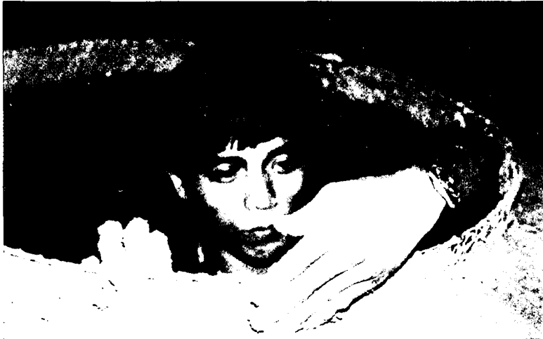
Plastering the man-hole of a-2000 liter water tank, Asian Institute of Technology, Bangkok, Thailand.
