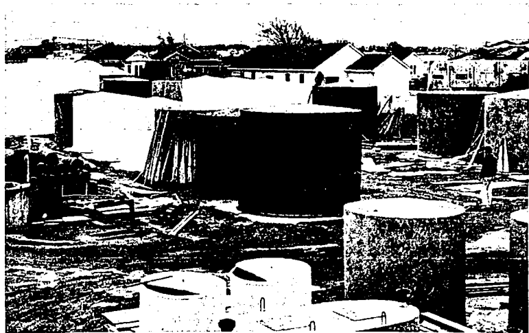
Typical ferrocement tank manufacturer's yard in New Zealand. Over 50 manufacturers build tanks in the capacity range 200-5000 gallons.
