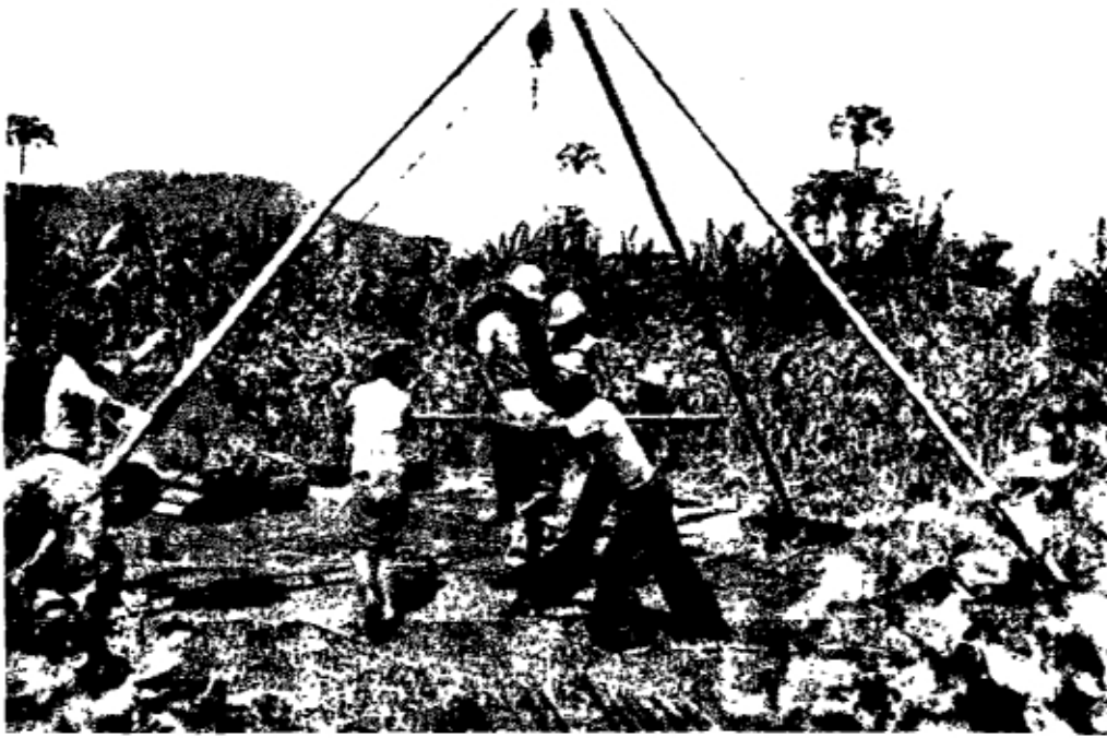
Fig. 3b. Hand drilling showing tripod support.
