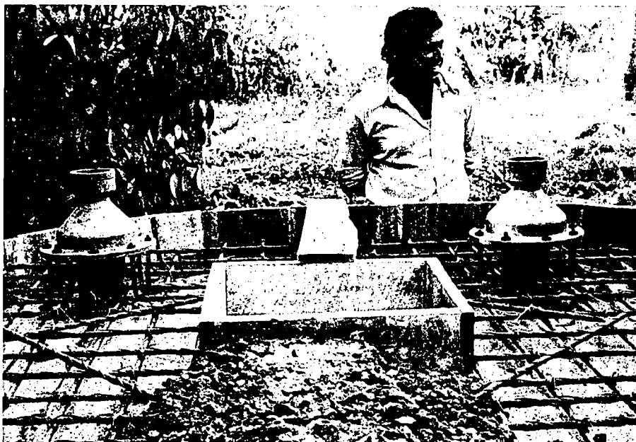
FIGURE 18. SLAB FOR AID HAND PUMPS (SRI LANKA)
