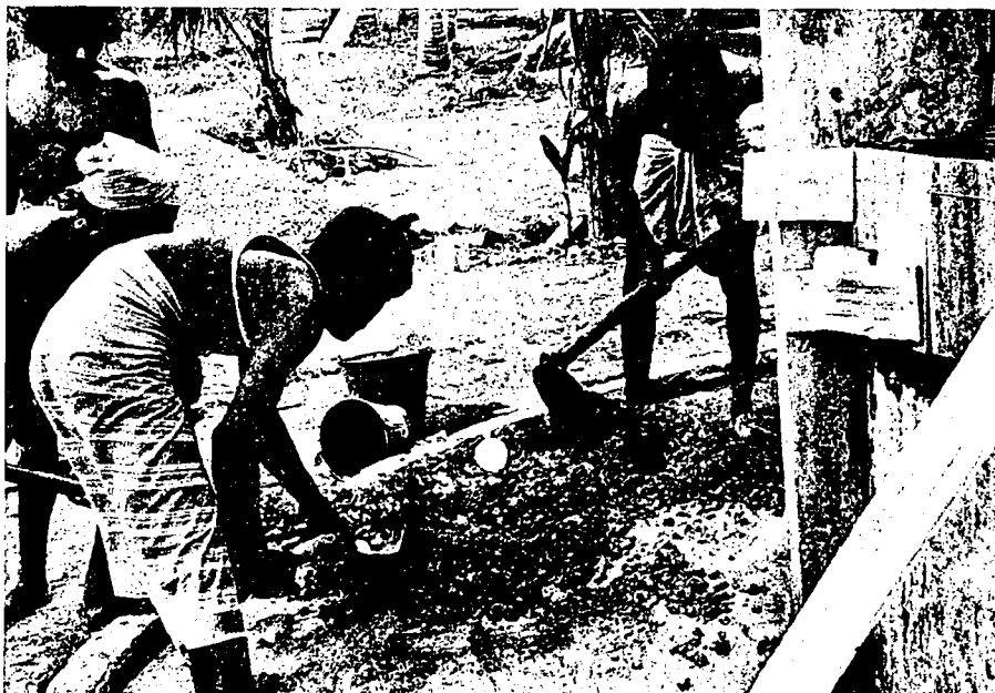
FIGURE 17. SERUPITA, SRI LANKA VILLAGERS HELP DEVELOP AN EXISTING WELL FOR INSTALLATION OF TWO AID HAND PUMPS
