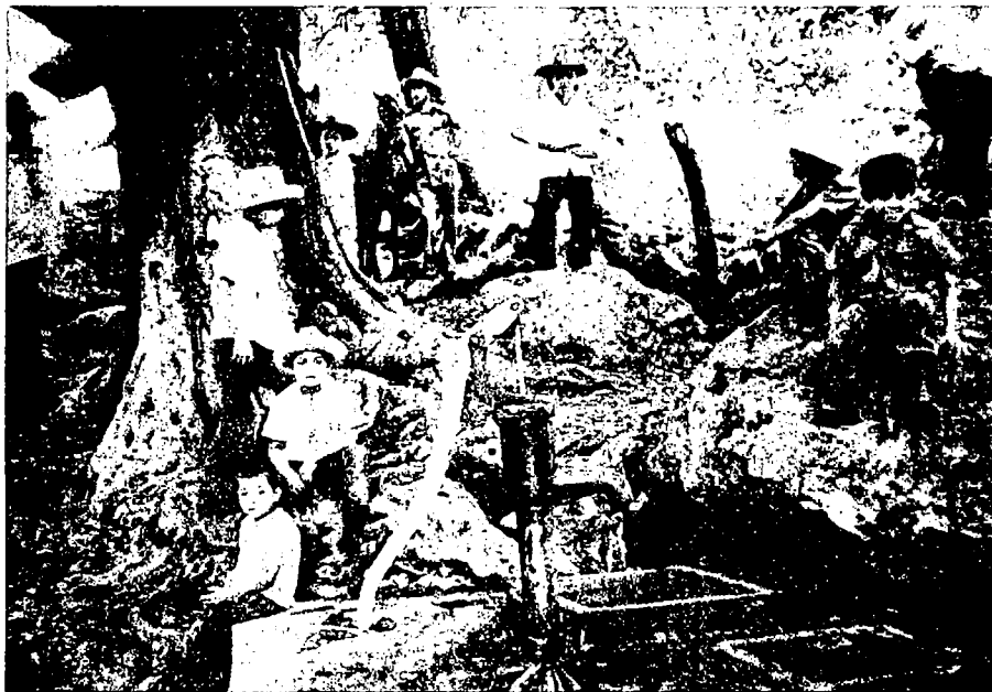
FIGURE 4. AID SHALLOW-WELL MODEL HAND PUMP (NICARAGUA)
