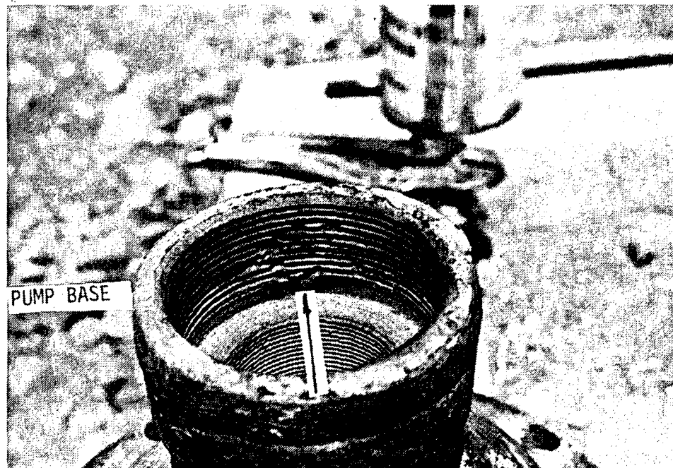
Another site with the porosity problem on the upper threads of the pump base. This causes excessive water leakage.
