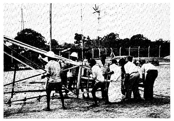
The installation of a  $\emptyset$  5 m windmill in Colombo, Sri Lanka; in the background the  $\emptyset$  3 m WEU-I windmill.
