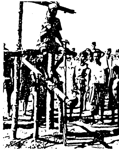
Fig.7.7 BAMBOO SCAFFOLDING, PIVOT AND LEVER USED IN DRILLING BY THE SLUDGER METHOD. (From "Jetting Small Tubewells By Hand," Water Supply and Sanitation in Developing Countries , AID-UNC/IPSED Item No. 15, June 1967.)
