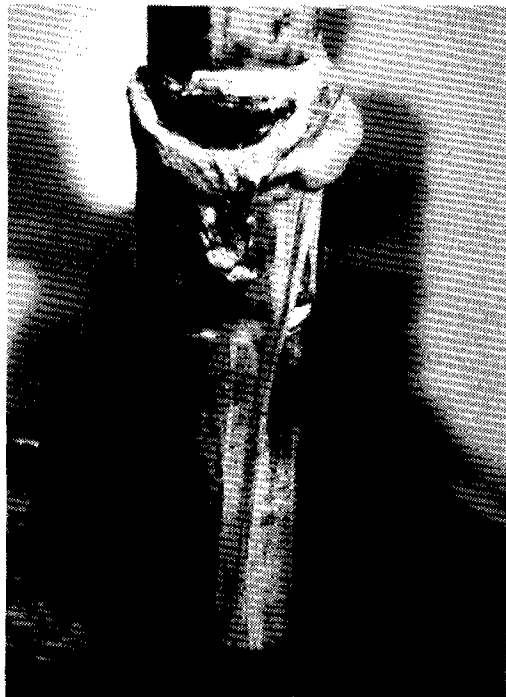
Figure 4.9 Fungus on the galvanized pipe of a handpump
