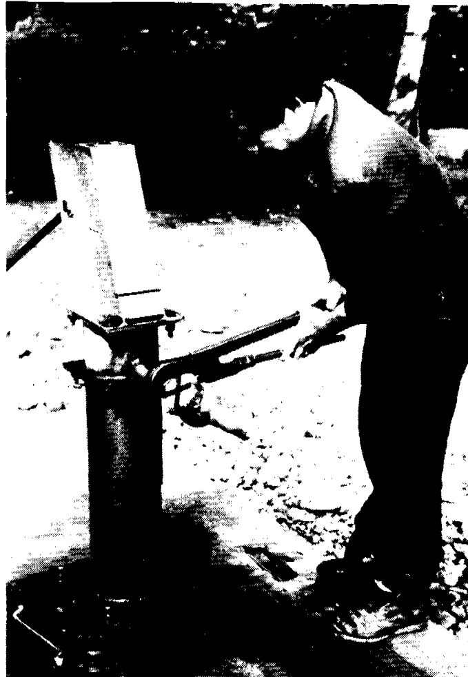
Figure 4.1 Well pad and pump stand of an India Mark II pump colored red-brown by corrosion products (southern Ghana)
