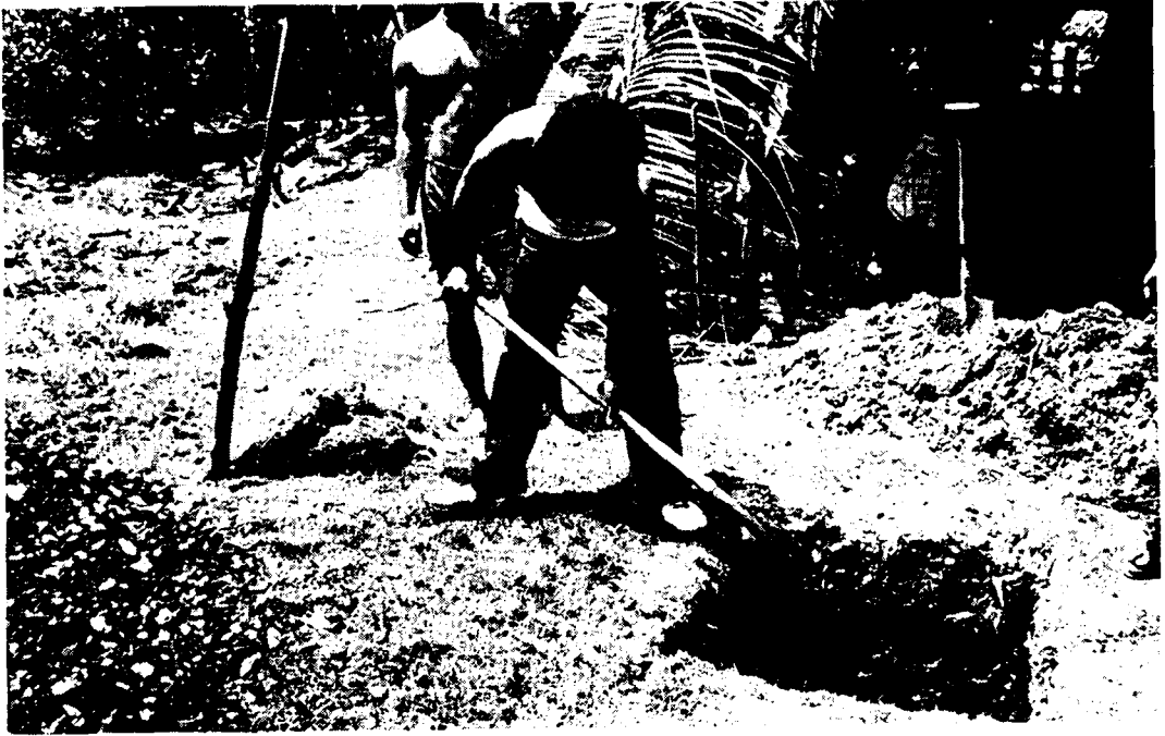
Figure 15. Backfilling with aggregate, step 1. Place about 6 inches of aggregate in the bottom of the well.
