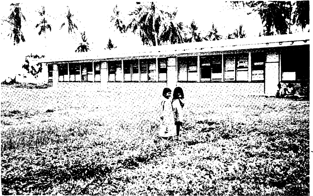
Figure 11. Typical site for "WERI WELL" installation.
