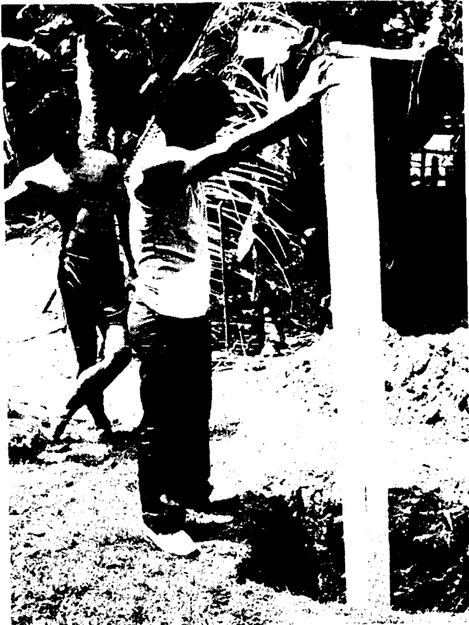
Figure 16. Placing the well casing. Place the 6-inch PVC pipe in the center of the well. This pipe will serve as the well casing.
