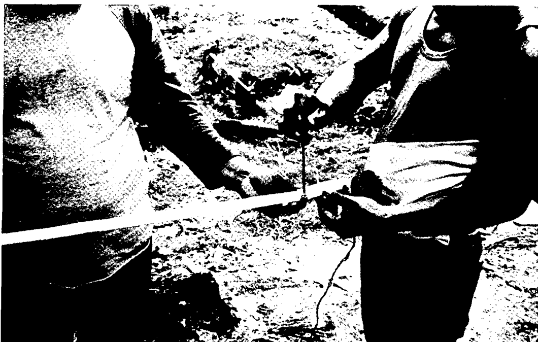
Figure 22. Connecting the well pipe and hose. Use another hose clamp to connect the other end of the rubber hose to a 10-foot length of \frac{1}{2} -inch PVC pipe (the well pipe).
