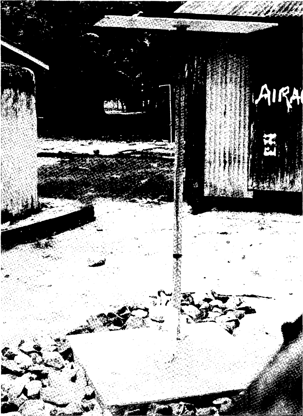
Figure 1. A completed "WERI WELL" installation.
