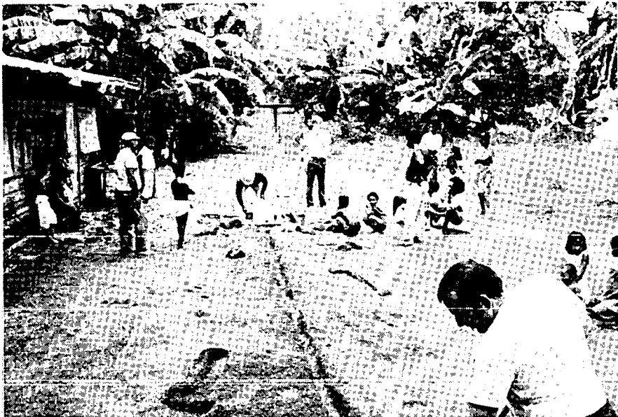
Figure 36. Running the \frac{1}{2} -inch PVC pipe. Run pipe from the well to the tank location. The pipe should be buried slightly below the ground to help protect it from damage.
