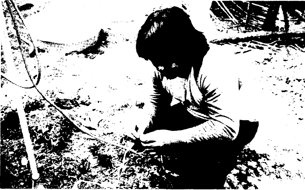
Figure 33. Connecting the wiring, step 2. Connect the white wire from the solar panel cord to the white wire from the pump cord by twisting them together. Do the same for the dark wires.
