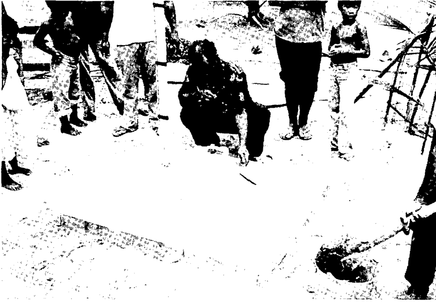
Figure 37. Pouring the slab. Use the 2-inch by 4-inch lumber to make a 4 feet by 4 feet form around the well, mix concrete, and pour into the form.
