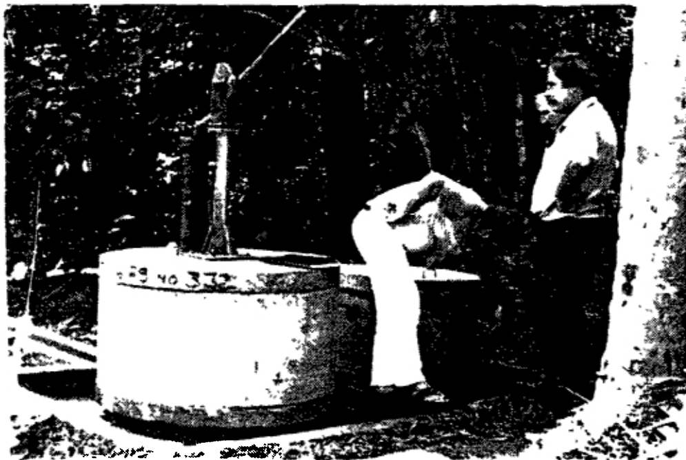
FIG4.8 EARLY FINNISH IRON REMOVAL PLANT
