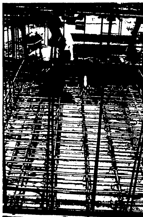
Fig. 3.12 Structural Frame of Filter Walls
