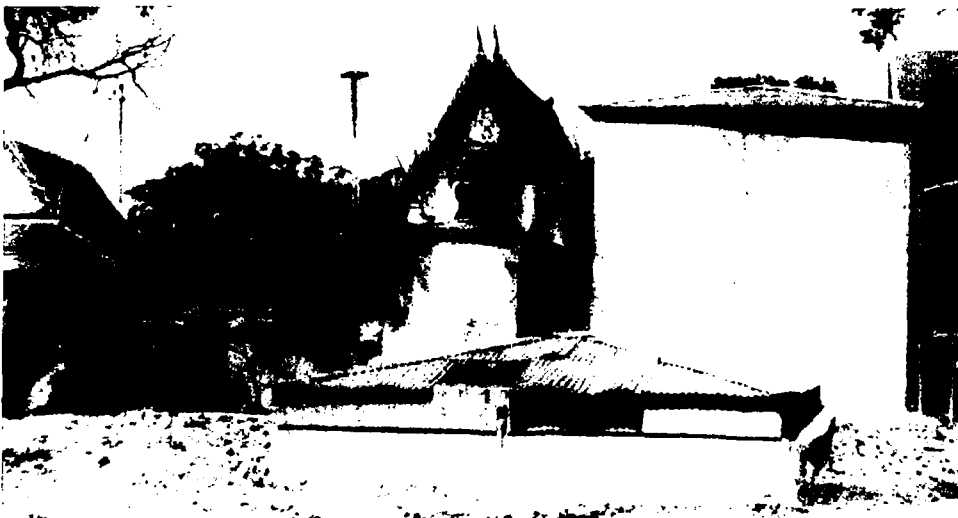
Fig. 3.22 Covering of Water Treatment Plant
