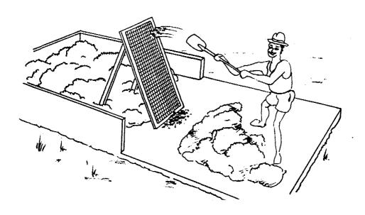
After drying the sand in the sun, pass it through a sieve of 6 mm mess to remove gravel, wooden chips and other coarse material.
