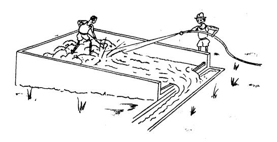
Direct a hose on the scrapings, and move them about. Sand will settle, and the water containing the impurities will overflow the weir and will be removed. Stir the sand while washing to help wash out the dirt.
