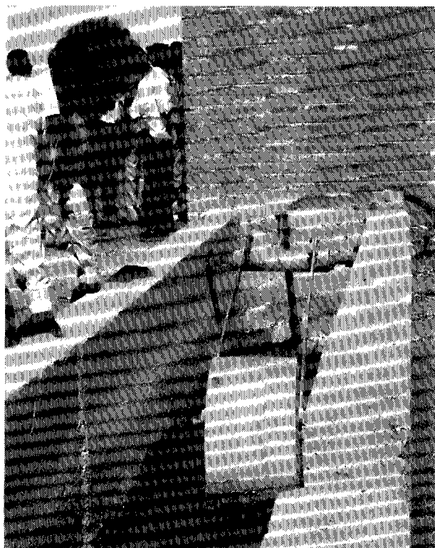
Figure 10.4: Float valve for constant water level, Gezira, Sudan 1983
