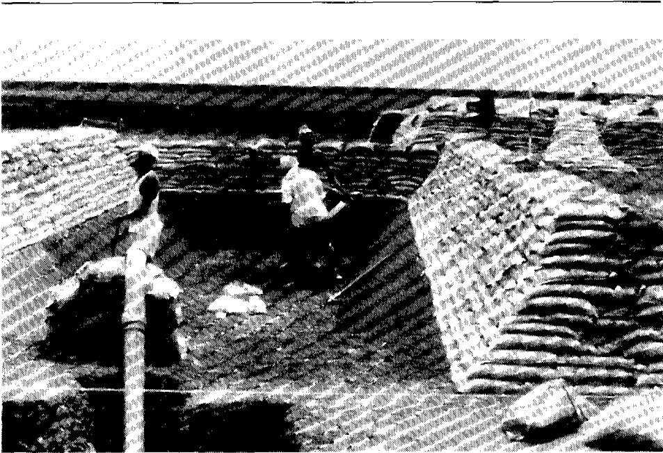
Figure 2.2: Horizontal flow-roughing filter under construction, Fau, Sudan (photo IRCWD)
