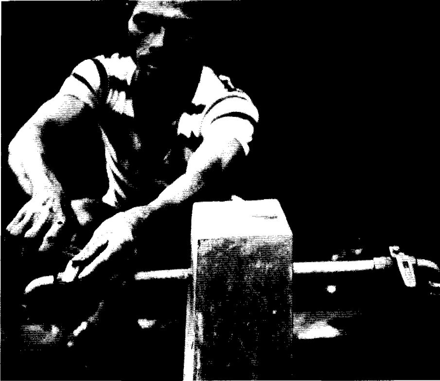
A local mechanic in Playangan, Indonesia, repairing a communal tap. Photo: PSWS Project Indonesia/Parwoto.
