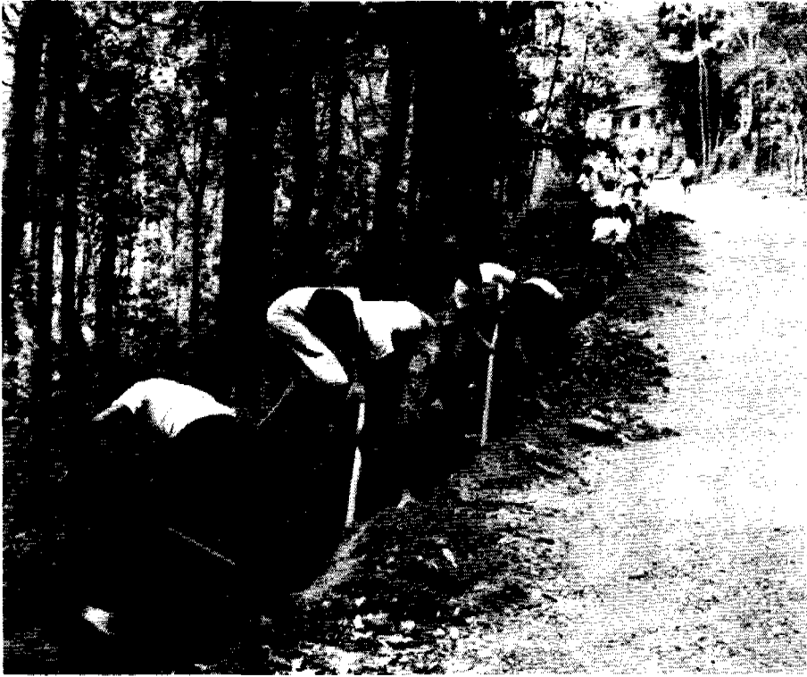
Trench construction involving the community. Photo: PSWS Project, Sri Lanka.
