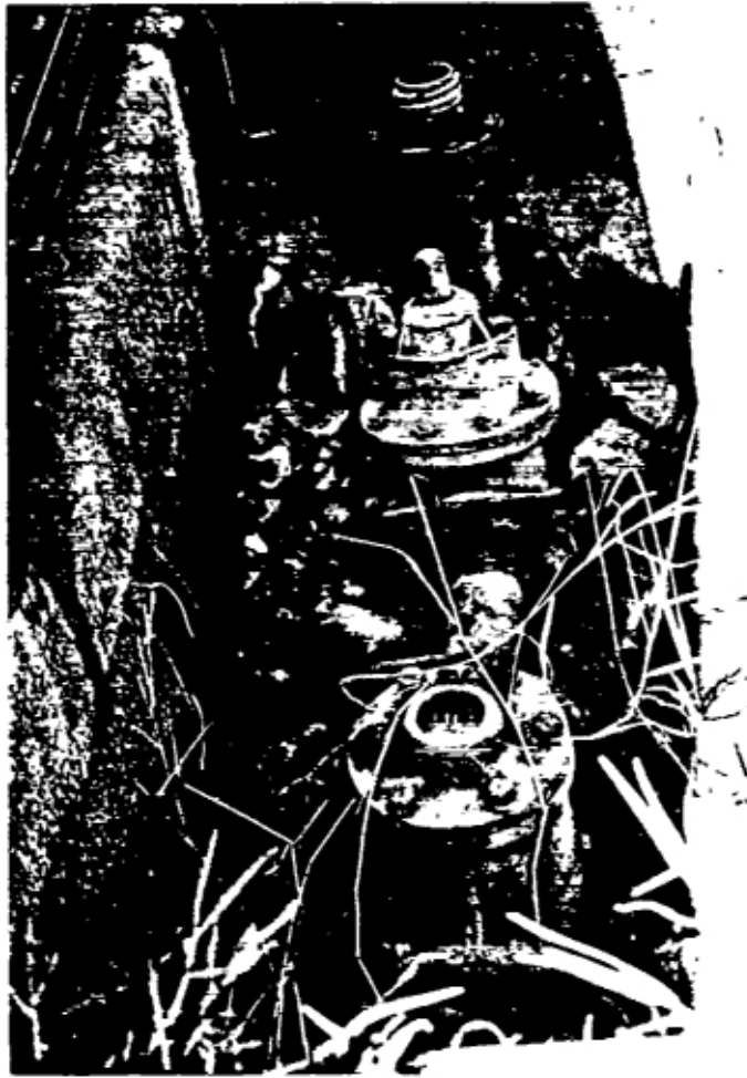
Figure 7. Condition of an unprotected metered fire hydrant in Addis Ababa, December 1989.
