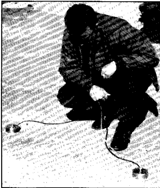
Listening for leaks with a geophone. (Courtesy Health Consultants, Inc.)
