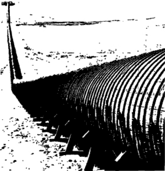
figure 4, Continuous woodstave pipe
