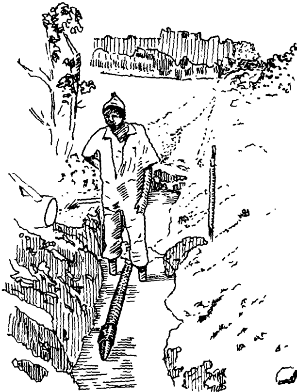
figure 21. Repair of bamboo pipeline.
