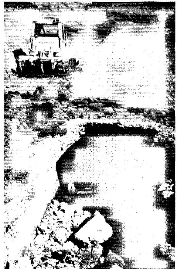
Unearthing the creek (Photo courtesy of Wolfe Mason Associates)
