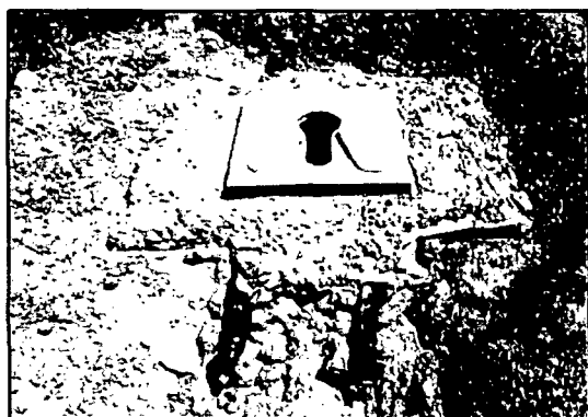
Figure 5.12 The squatting plate and SanPlat in position
