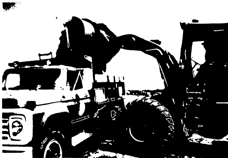
Figure 10–21.—Stockpiling soil, Waukegan, Ill.
