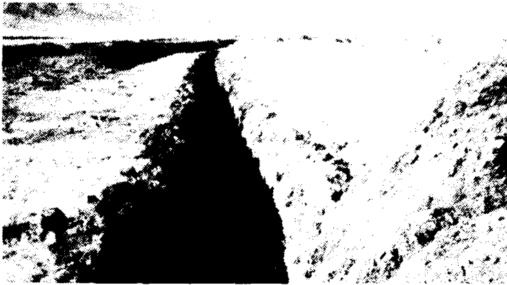
Figure 10-4.—Narrow trench operation.
