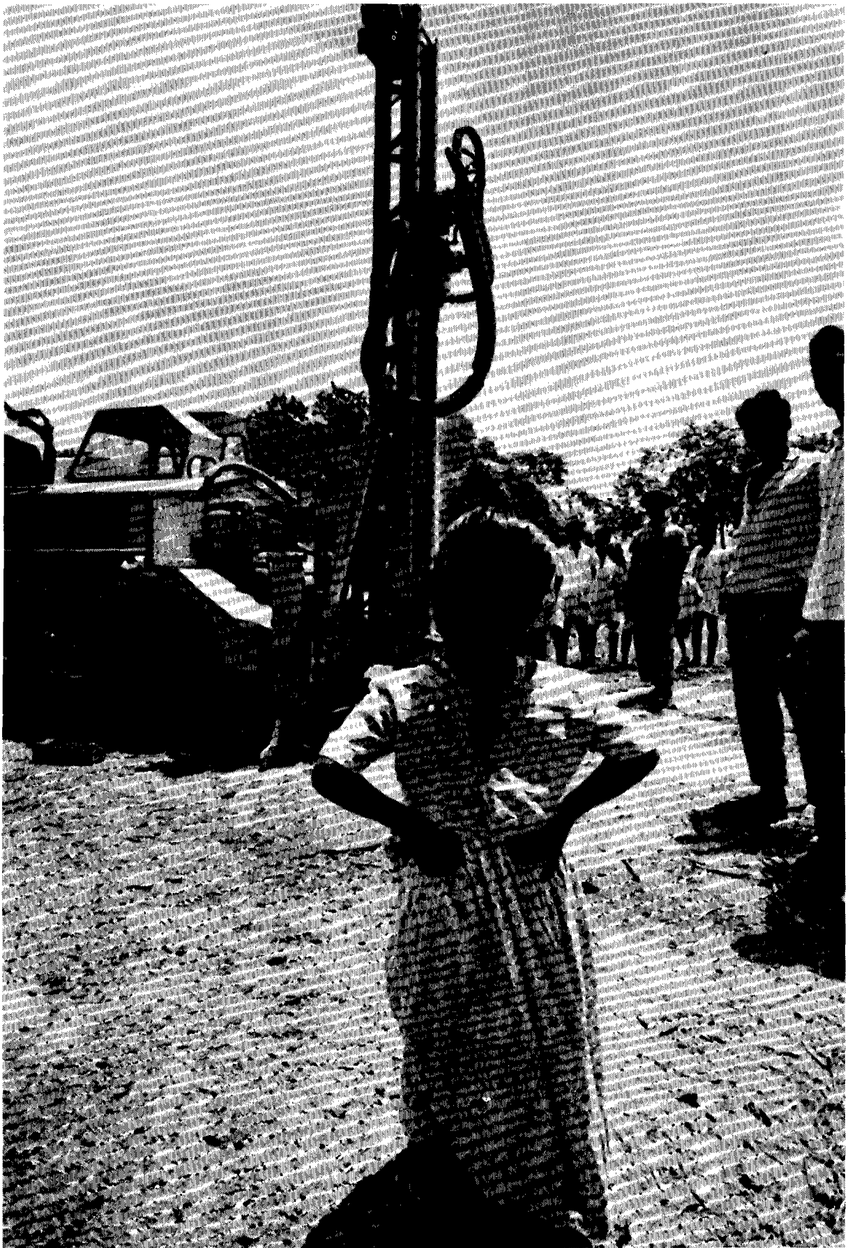
Bits of rock fly up as pneumatic drill bores more than 100 feet deep through solid rock (India; UNICEF photo by J. Blacomb).
