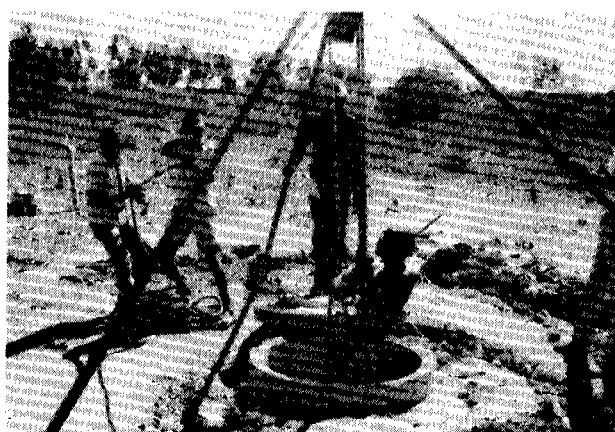
Hand-digging of a well
