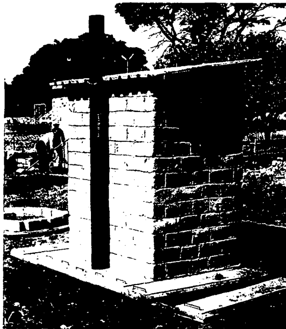
FIGURE 7: VIDP latrine built of sand/cement blocks
