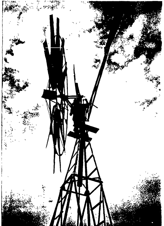
19. Playangan: the windmill with broken transmission
