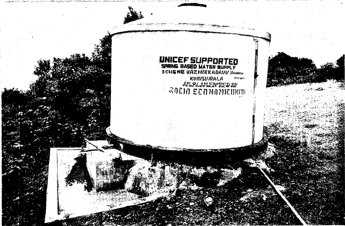
Ferro Cement Tank
