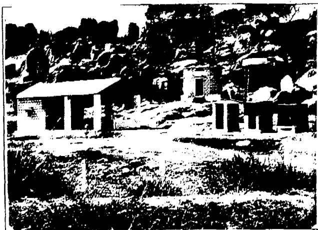
OVERALL VIEW OF RSSPC
