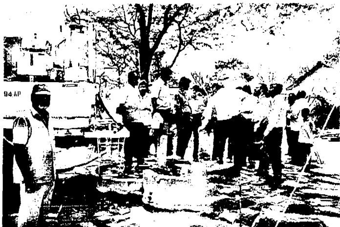
Hydro-fracturing Unit in use
