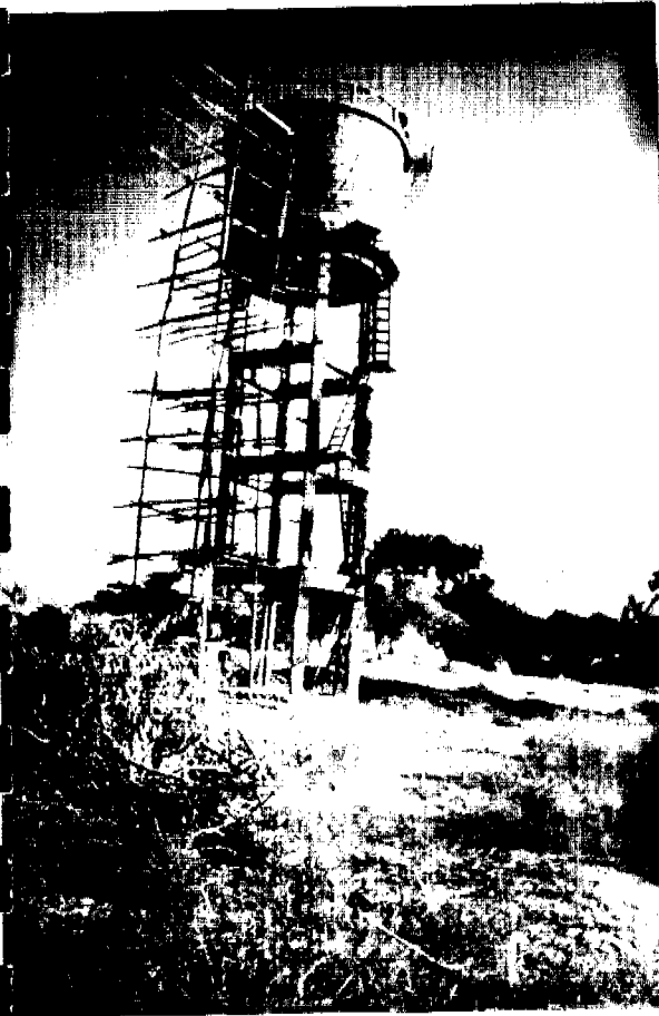
FINISHING TOUCHES AT SOGANUR OHSR (TOP)
