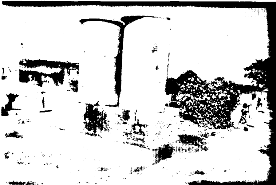
← CISTERN AT SAJEEVAPURAM WITH LEAKING BOTTOM & NO PLATFORM
