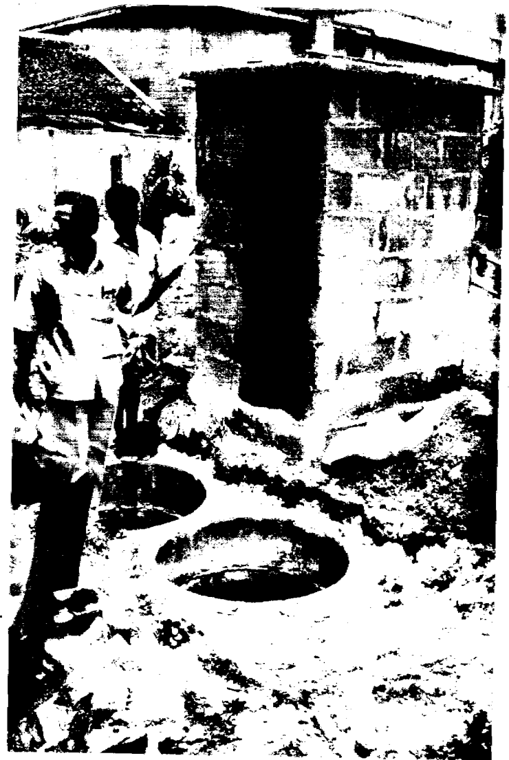
SST ABPALEM (AUG, 95) BREACHED BY EXCESSIVE RAIN WATER
