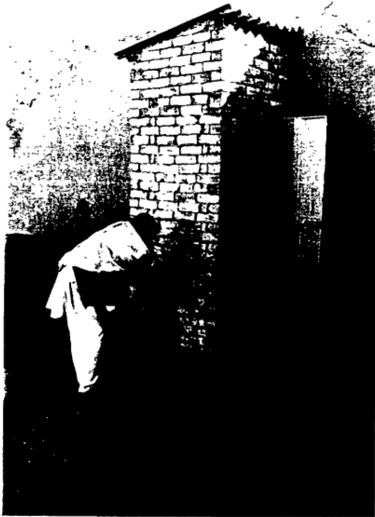
◀ Photo 9 Completed twin pit pour-flush latrine
