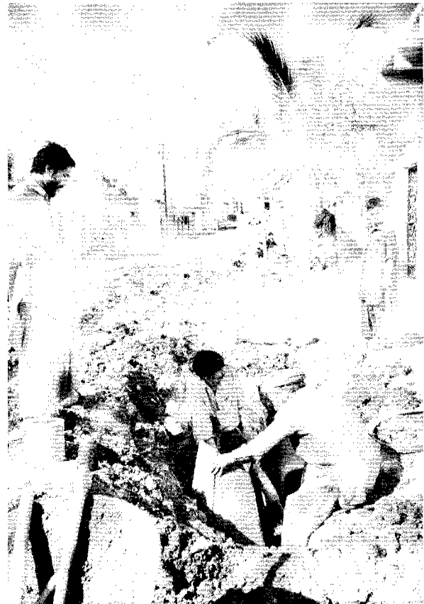
Rectification of large secondary sewer in Gulshan-e-Behar – Nazim's work.
