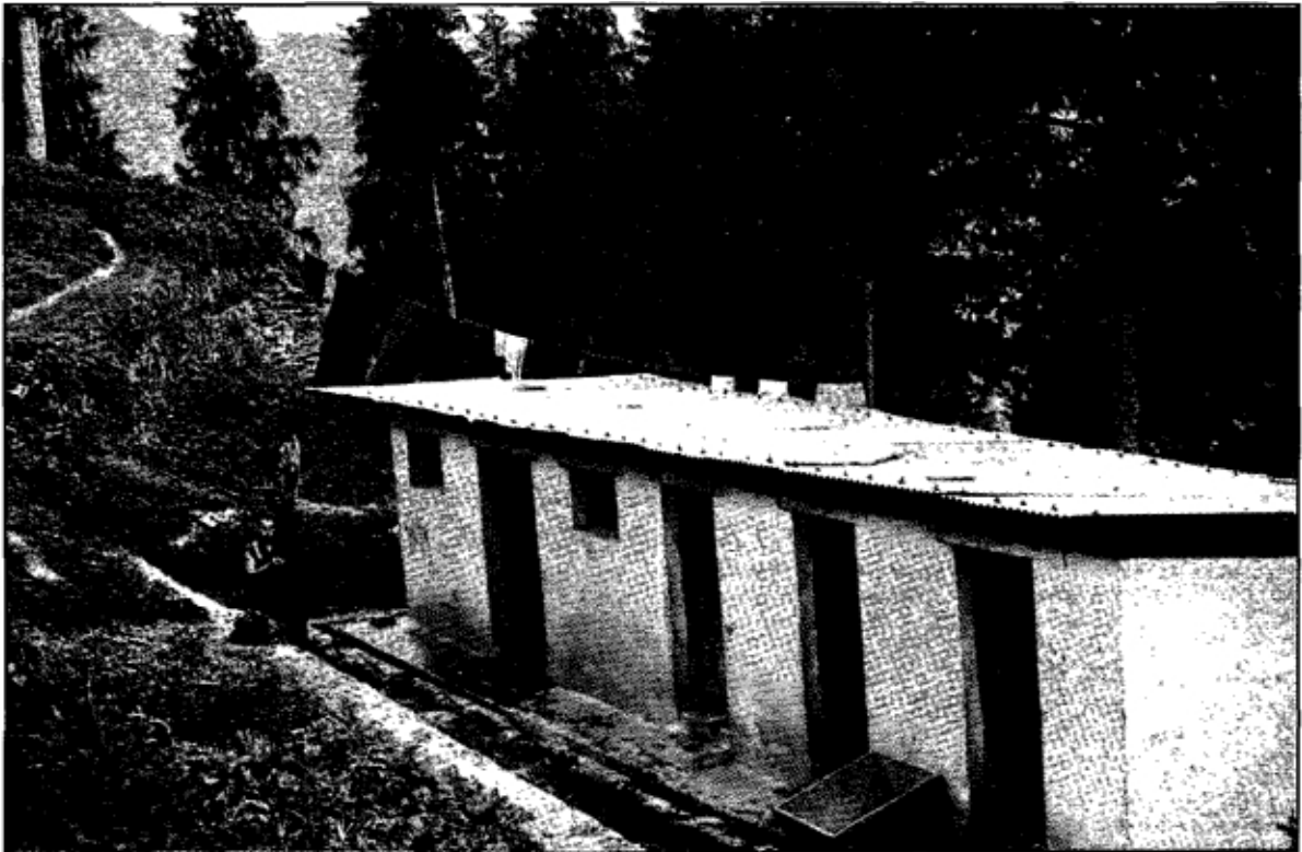
Recently constructed teachers toilet at Dechenphodrand Monastic School
