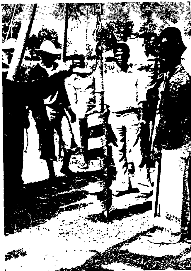
Construction of a hand drilled well.
