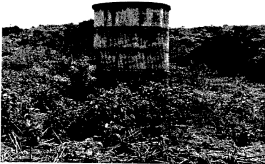
Abandoned communal water point, Uyoma Water Supply; Rarieda Division.
