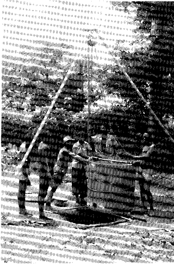
Lowering a filter ring into the hole.
