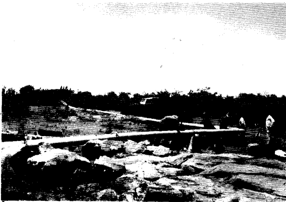
Figure 3.5 Steel pipes (G.I.) on rocky areas
