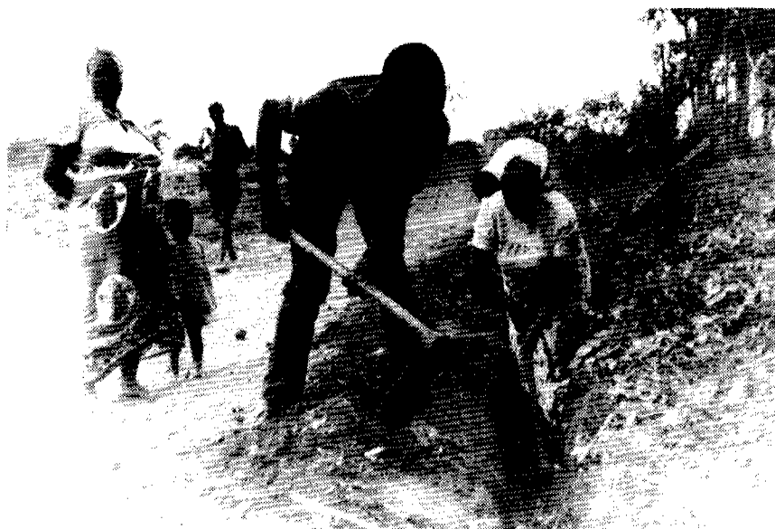
Figure 6.1 Community members digging trenches for a piped scheme
