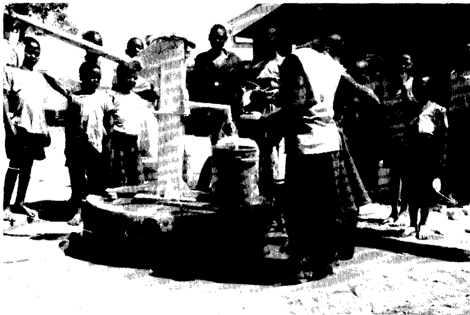
Completed community well
